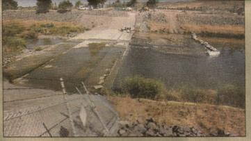
The Alameda County Water District is modifying the foundation of a rubber dam along Alameda Creek in Fremont to allow fish to pass through the area under low-flow conditions.
